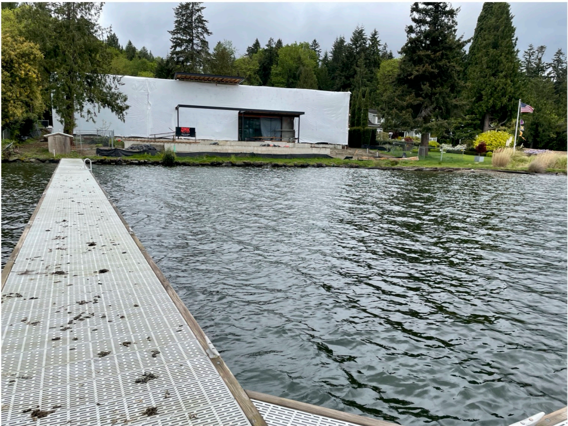
Photo 2 - Existing dock looking landward.
