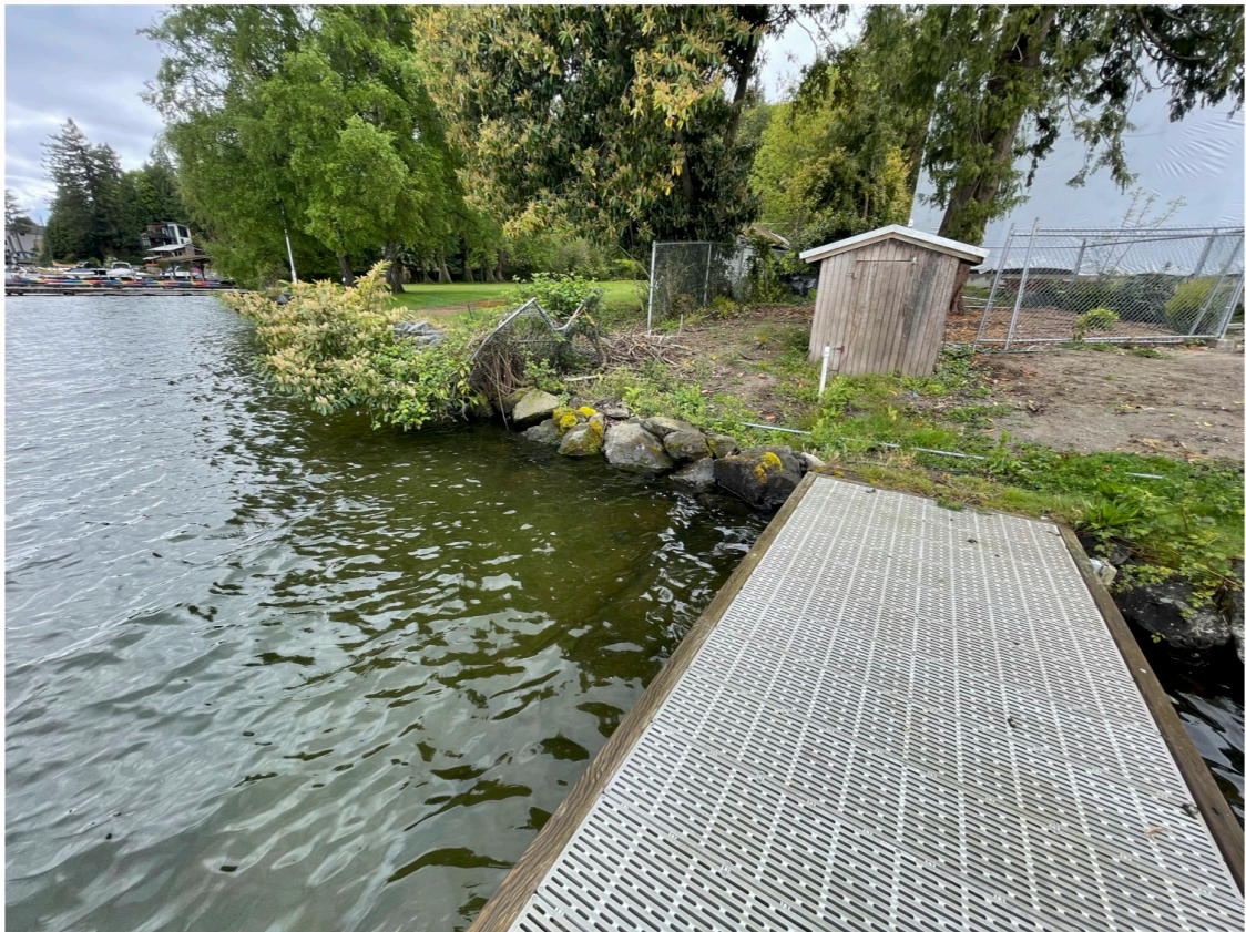
Photo 4 - Existing shoreline looking south.
