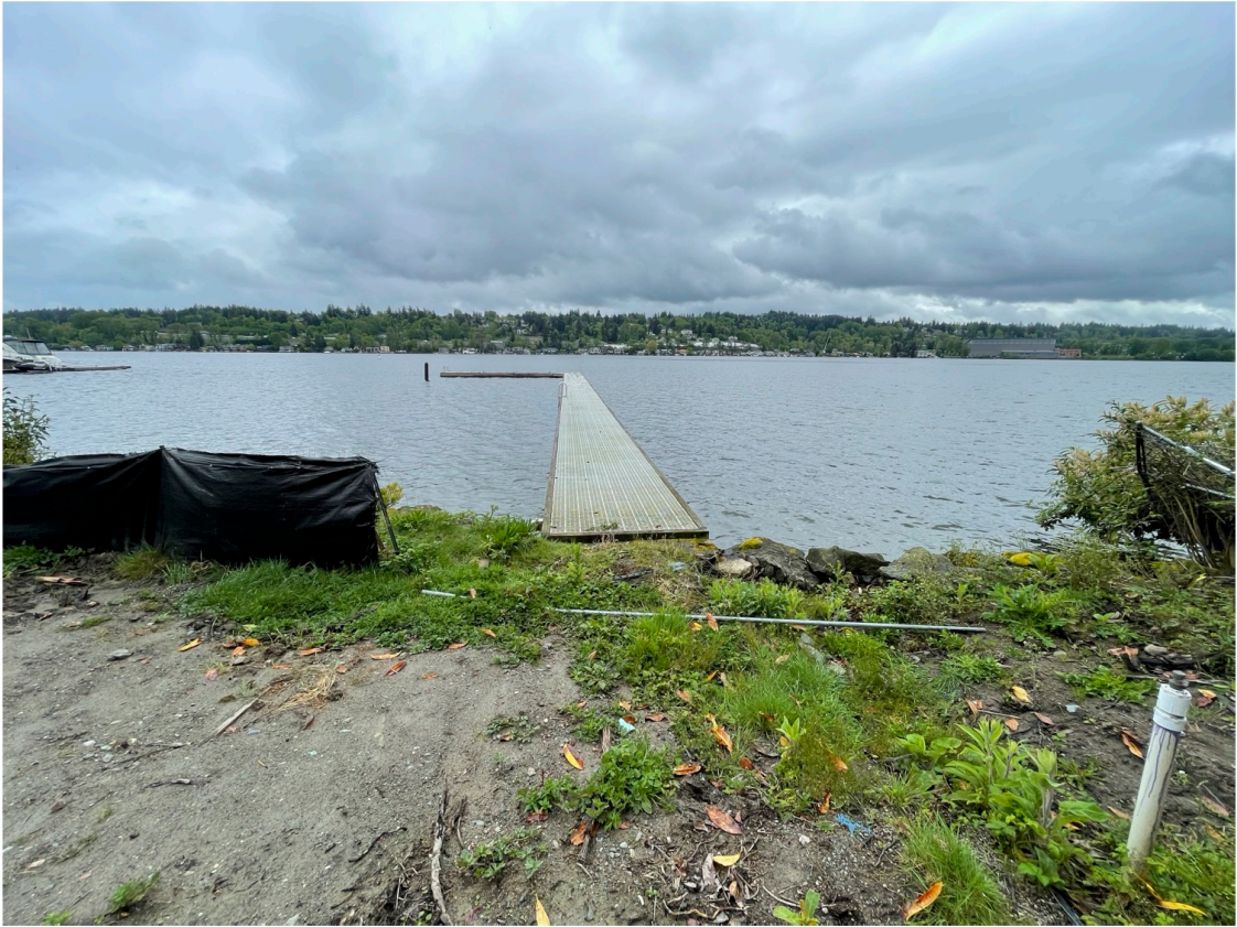
Photo 1 - Existing dock looking waterward.
